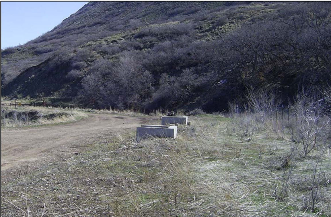
In 2004 external funding was used to upgrade this section of canal to a covered concrete box.
