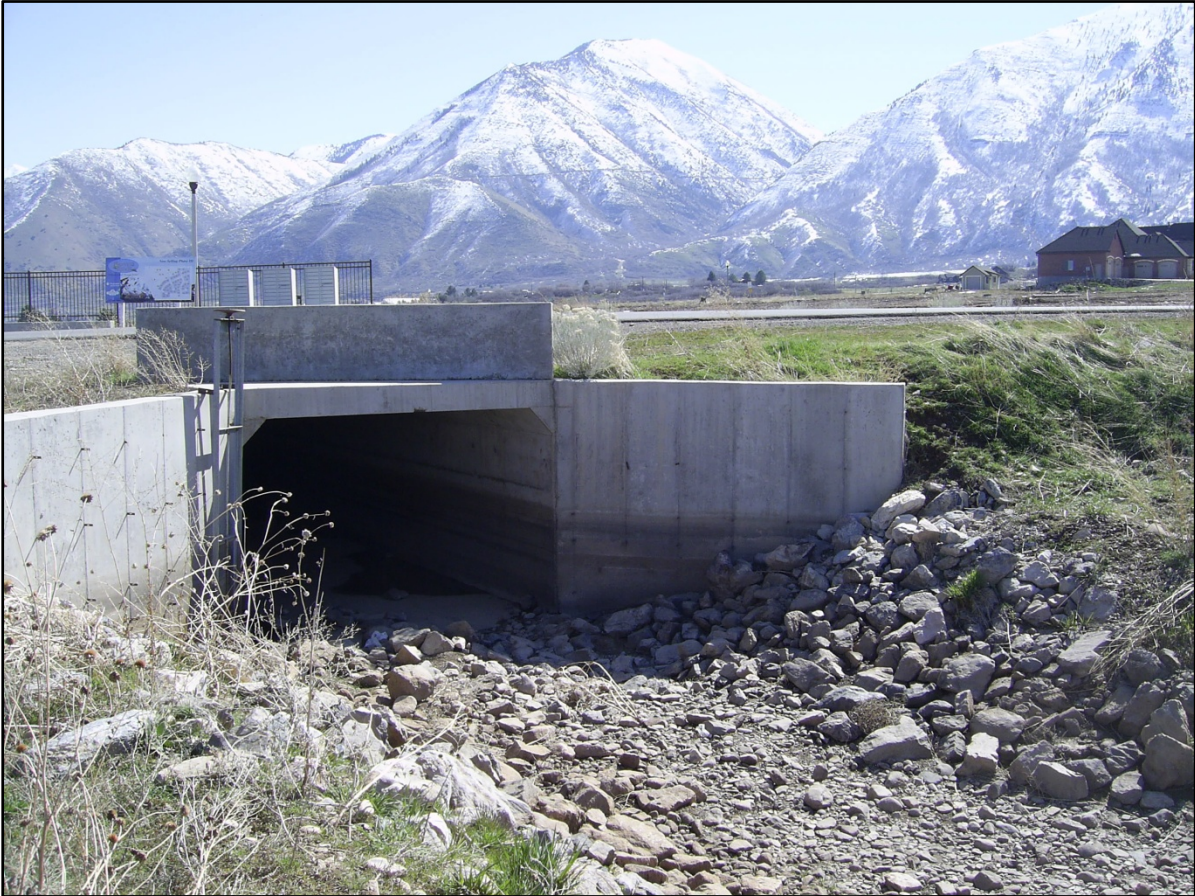
County roads that are built without a curb and gutter allow storm water to enter the canal.
