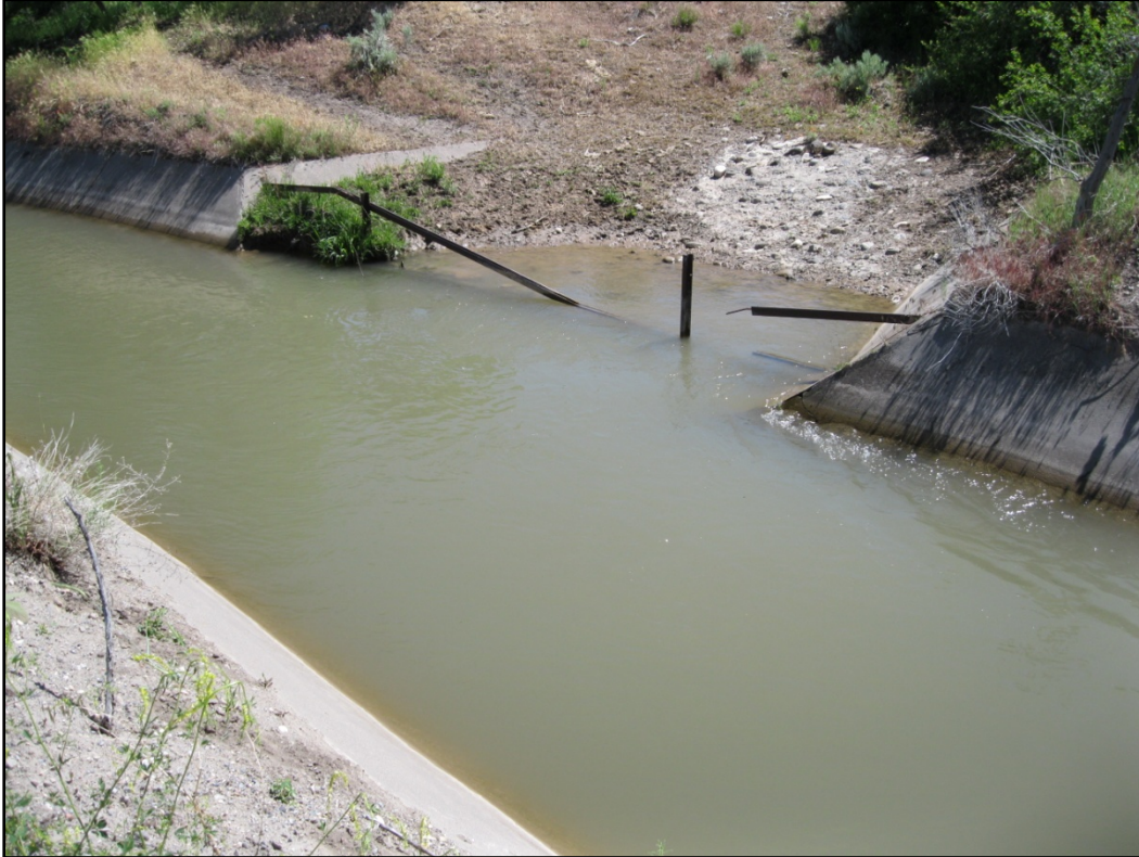
Animal watering point on the uphill side of the Strawberry High Line Canal.
